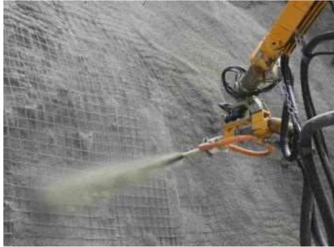
Figure 6. Spraying concrete (idn.sika.com)
