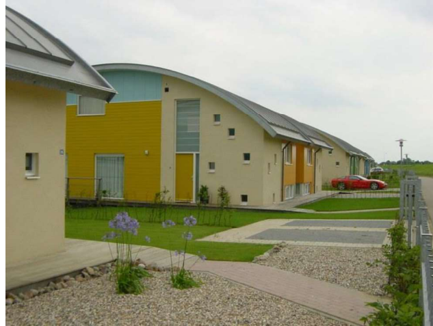
Figure 2: Amphibious housing (Maasbommel, the Netherlands) (Source: Amphibious Housing in Maasbommel, the Netherlands — Climate-ADAPT )
