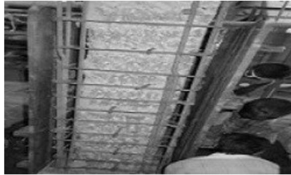
Figure 3. Shuttering adjustment.
