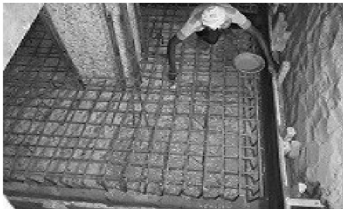
Figure 2. Application of Epoxy Bonding Agent.
