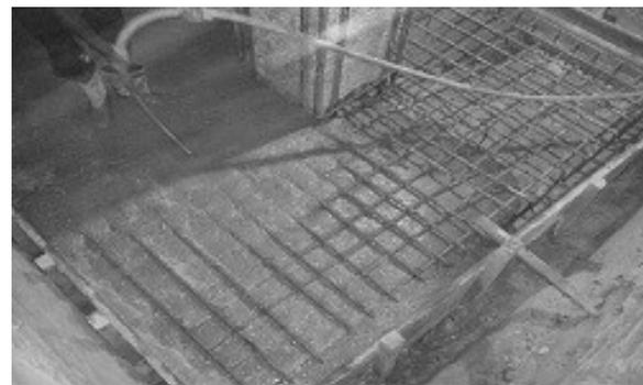
Figure 4. Pouring of Micro Concrete.
