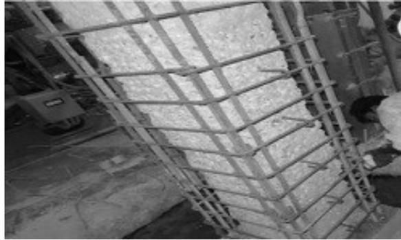
Figure 1. Additional Reinforcement Provided for Strengthening.
