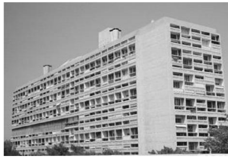
Figure 2. Unite d habitation of Marseille.
