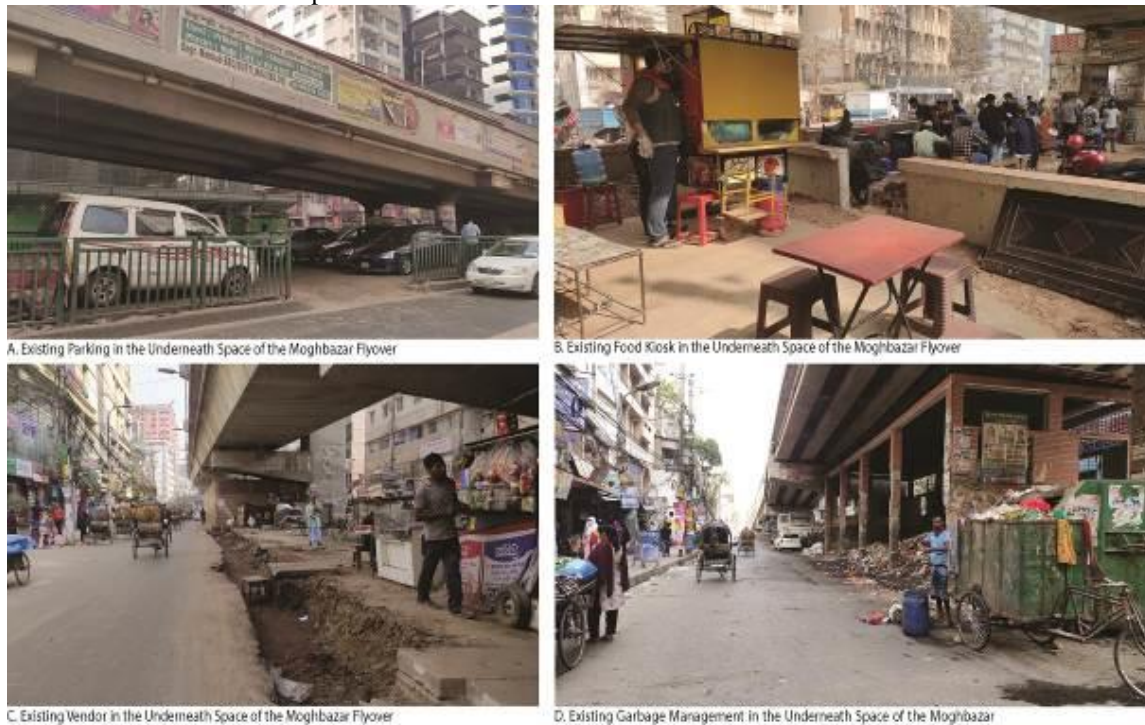
Figure 4: Photographed Functions Prevailing in the Underneath Spaces of the Moghbazar Flyover. Source: Photographic Survey.
