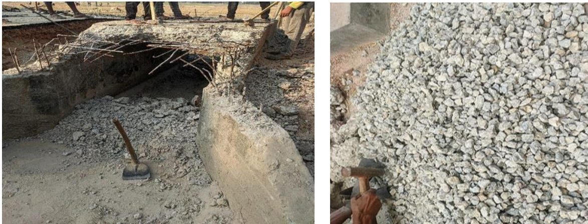
Figure 1. Collection of demolished concrete blocks and making of RCA
