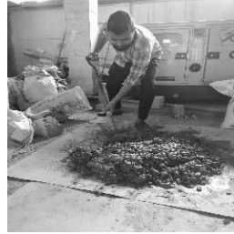
Figure 2. Concrete wet mixing
