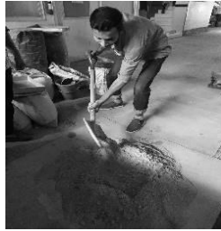
Figure 1. Concrete Dry mixing
