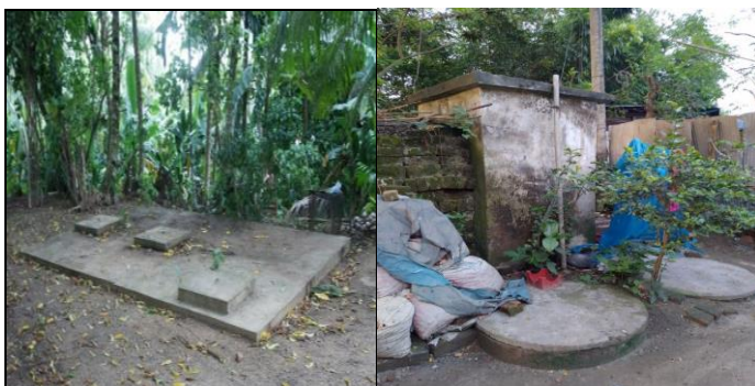
Figure 7. Picture of some accessible septic tank
