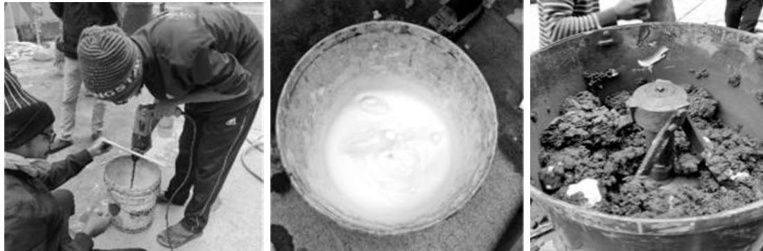
Figure 1. Manual generation of foam and mixing with composite mortar.
