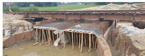
b) Complete rebuilding of a bridge (RCC box culvert)
