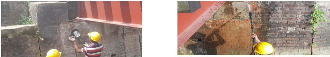
a) Scrapping, wire brushing etc. (B/N-131)
