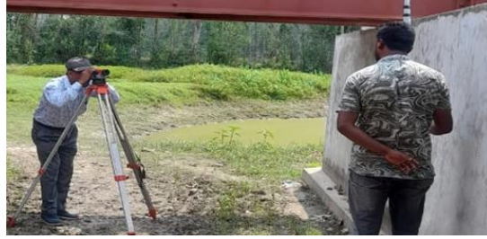
Figure 7 Measurement of Settlement of Bridge No. 131 (up) on 15.06.2023
