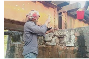
c) Bridge No. 131 (up)
