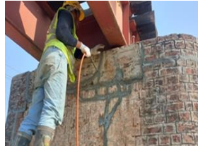
b) Bridge No.131(dn)
