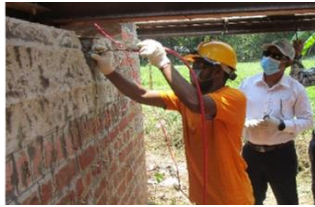
a) Bridge No. 111(up)
