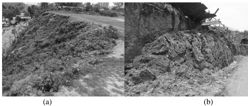
Figure 1: (a) Hill considered in this study, (b) current situation of the hill after landslide.
