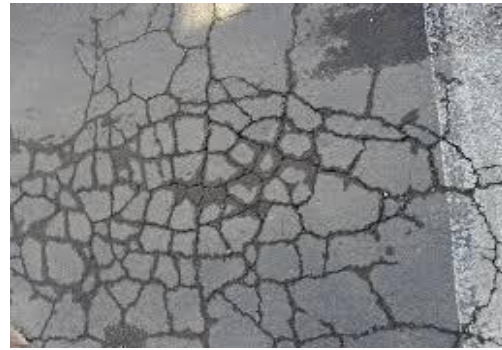
Fig 3: Fatigue cracking
