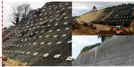
Fig: 1.5 Soil nails technique
